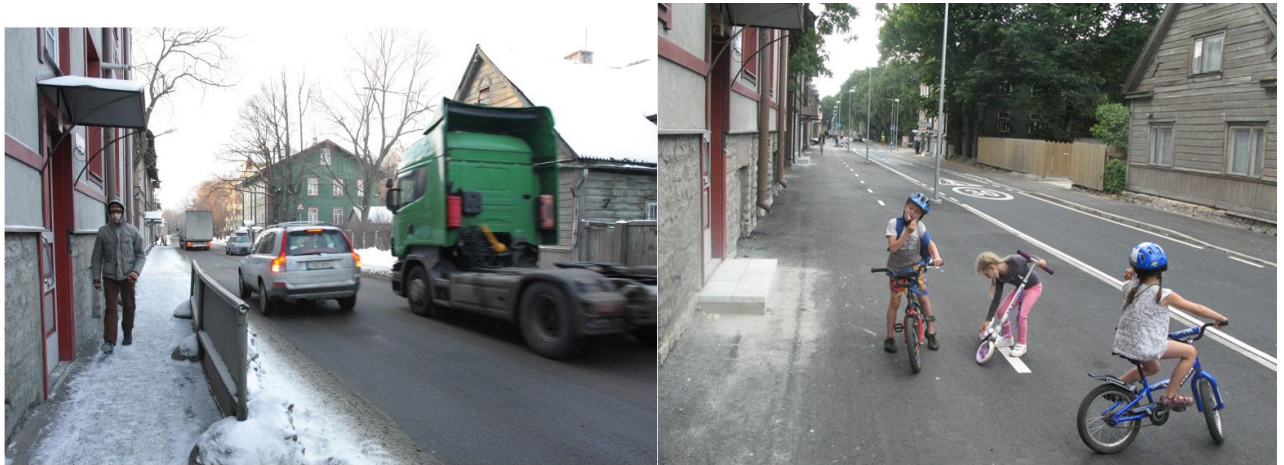
Figure 2. The city's main goal is to connect all existing bikeways into one safe network. Soo Street before and after reconstruction. Soo Street was built from the former two-lane street into one-way street with one lane. On the left side of the street the 4.5 meters wide bikeway was built and the sidewalk with the width of 2 meters on the right side of the street
