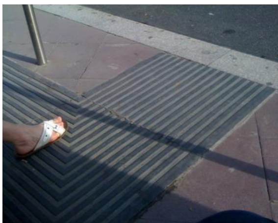
Figure 8. Embossed guide plate at a bus stop in Barcelona
