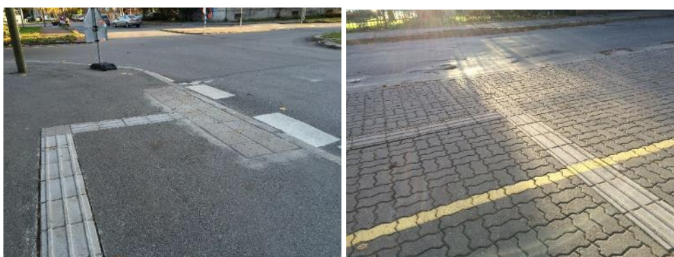
Figure 14. directing and warning tactile pavements in front of the building in 59 Endla Street
