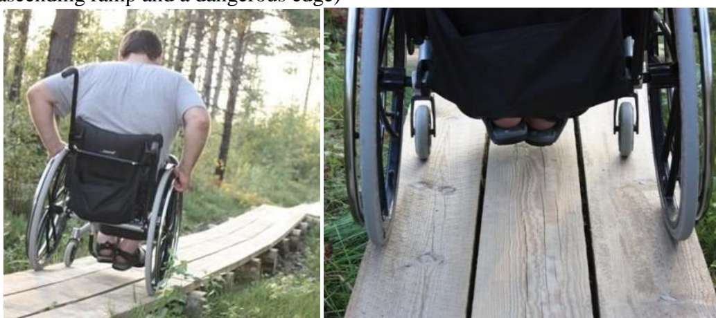
Figure 23. New beach road to the outdoor toilet in Pirita and an inaccessible disabled toilet (ascending ramp and a dangerous edge)
