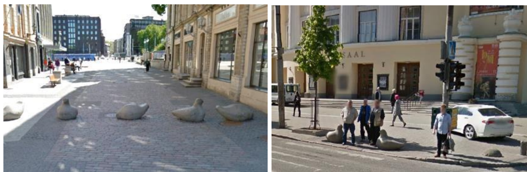
Figure 16. The concrete barriers on Harju Street are grey (poorly noticeable) and the space between them is sometimes too narrow (left image) for mobility equipment (electric wheelchair, scooter, etc.)
