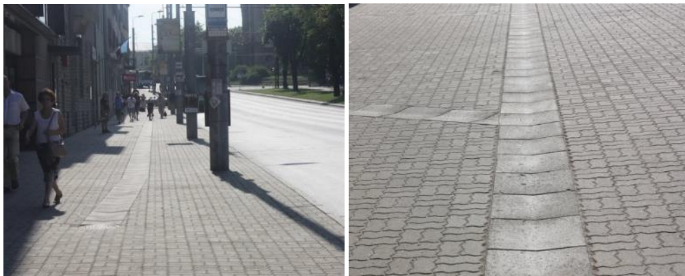
Figure 15. The sloping street gutters on Kaarli Puistee are perfect and not hindering for anyone
