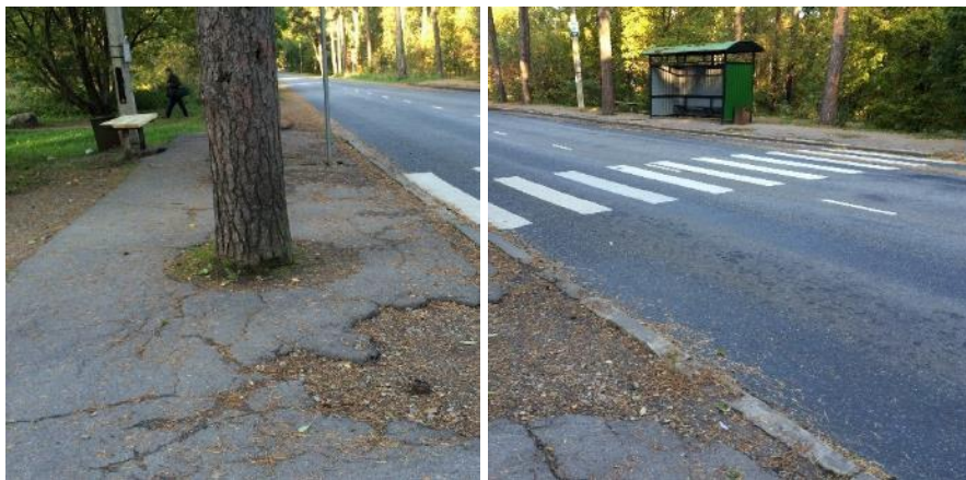
Figure 7. Urva stop in Maarjamäe: the curbstone of the pavement is 15 cm high, the asphalt has holes, unevenness, difficult access (Association of Persons with Mobility Disability in Tallinn)
